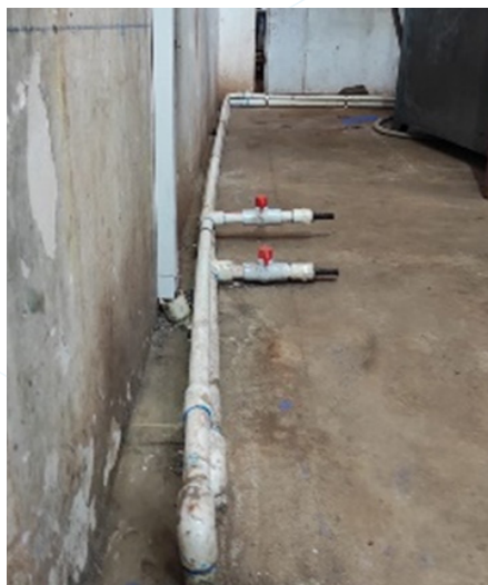
Providing Plumbing Connections
