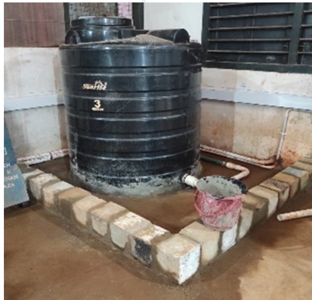
Providing water connection for the entire PPT lab.
